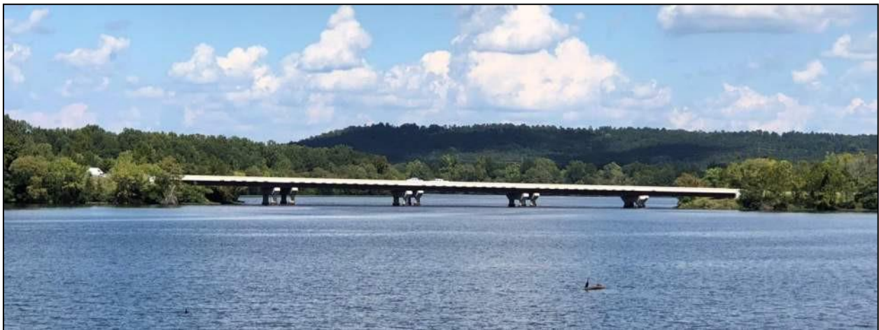
Figure 10. I-40 Bridges over Illinois Bayou/Lake Dardanelle, Looking North
