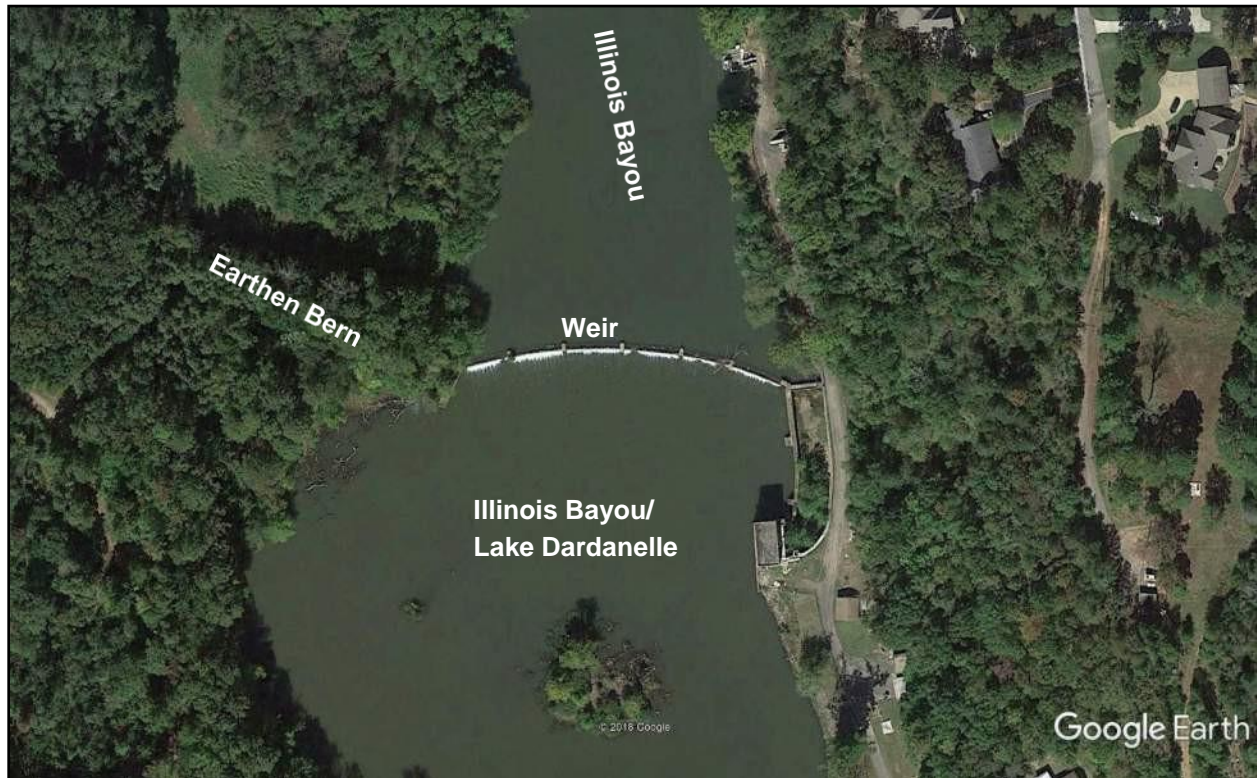
Figure 11. Low-Head Dam/Weir and Earthen Berm Upstream of RCC WTP
