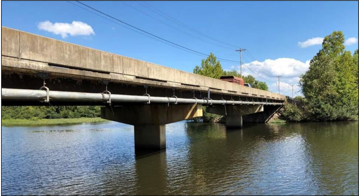
Figure 9. West Pleasant View Road Bridge Downstream Face
