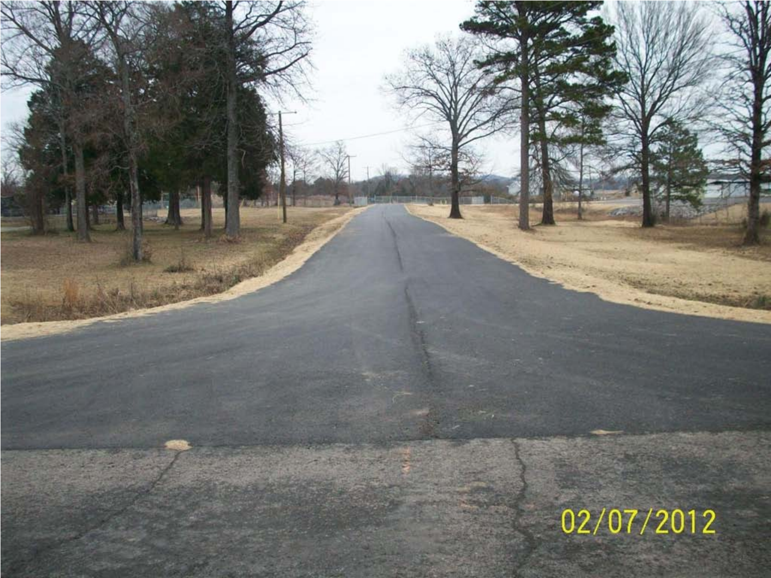
Access Road - After
