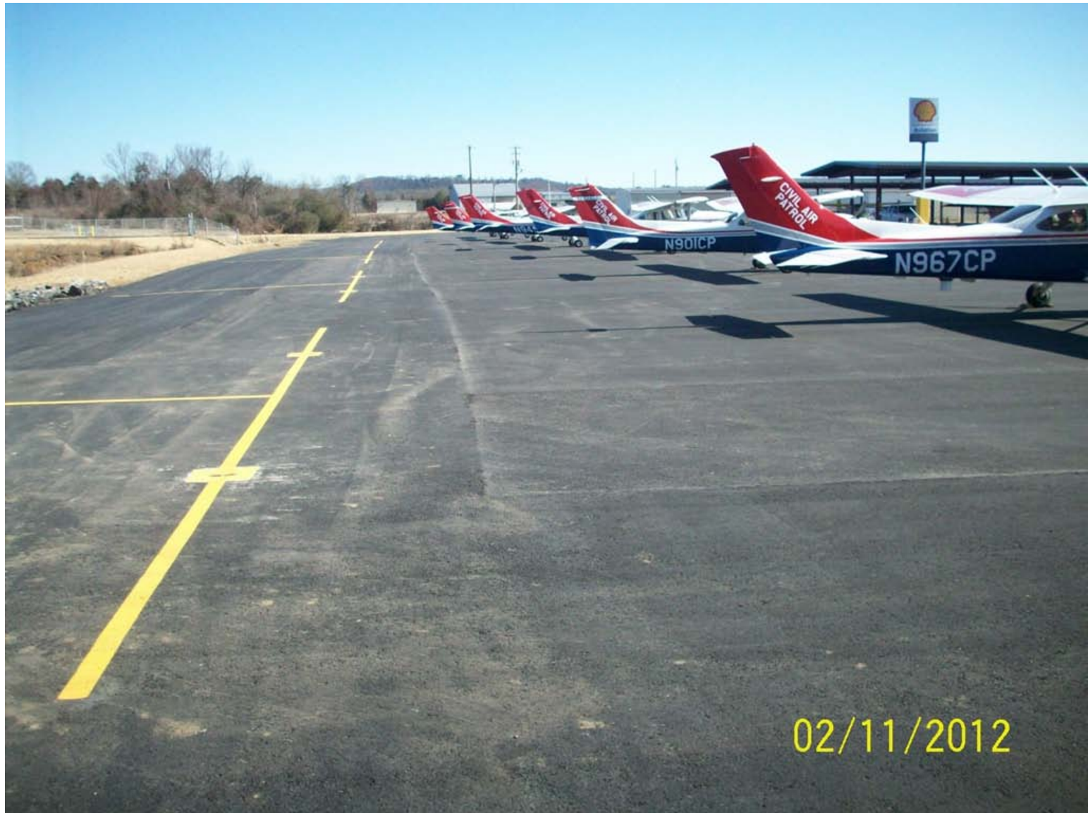
Ramp, North Edge - After
